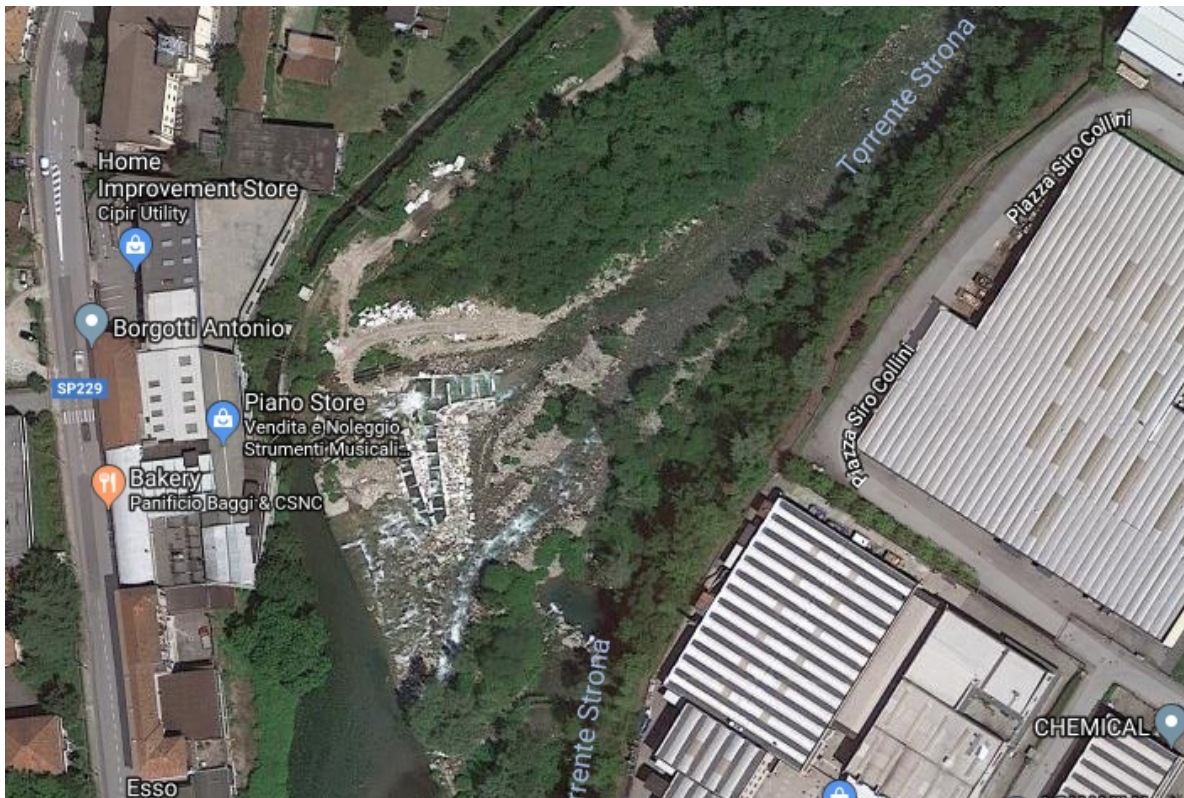
Figure 2. An aerial image of the weir and the fish-ladder in the Strona river.
